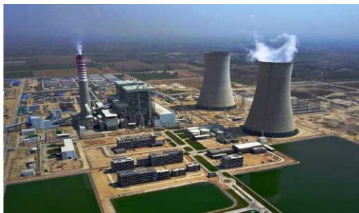
电厂 Power plant
